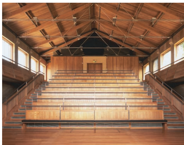
Right: Haberdashers' Hall, London. American white oak is used throughout. The ceiling diagonals are the top chords of the steel-tied roof trusses (see also back cover). Hopkins Architects. Engineer: Arup.
