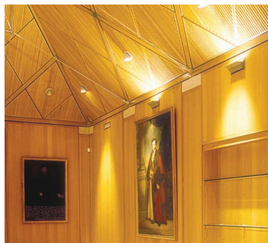
Far left: Queen's Building, Emmanuel College Cambridge, UK. The roof trusses use American white oak. Hopkins Architects. Engineer: Buro Happold.
