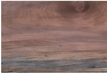
DECAY OR ROT: The breaking down of the wood substance by fungi. The discoloration of the sapwood indicates the initial evidence of decay.
