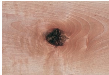
UN SOUND KNOT: A circular area that once formed the base of a branch or twig and has a pith centre. (In some cases the wood may be missing).
